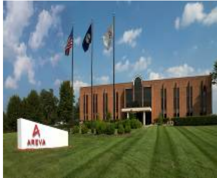
OFR Upgrade Expansion $37.7M
